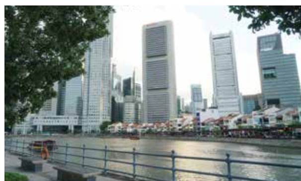
▲ Kantor Pusat OCBC Bank, Singapura OCBC Bank Head Quarter, Singapore
